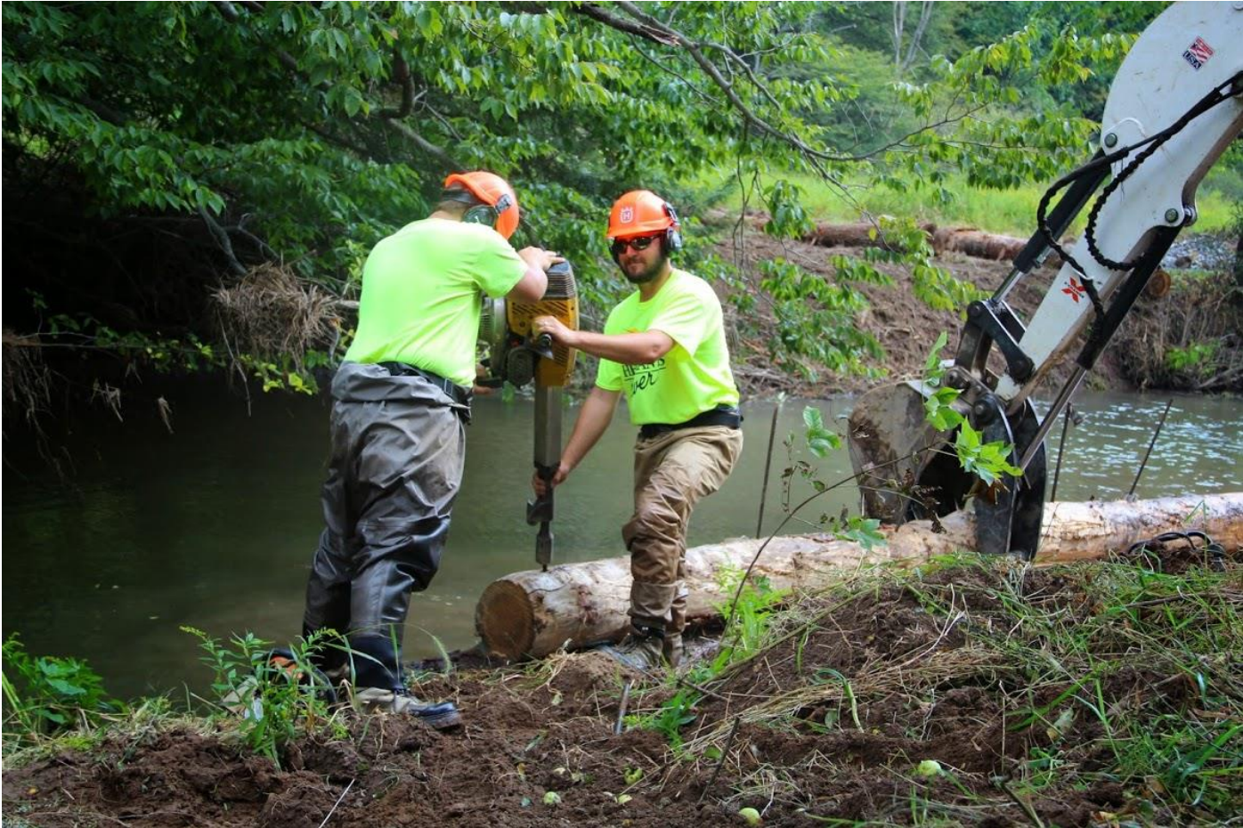
In-stream construction of mudsill overhead cover structure
