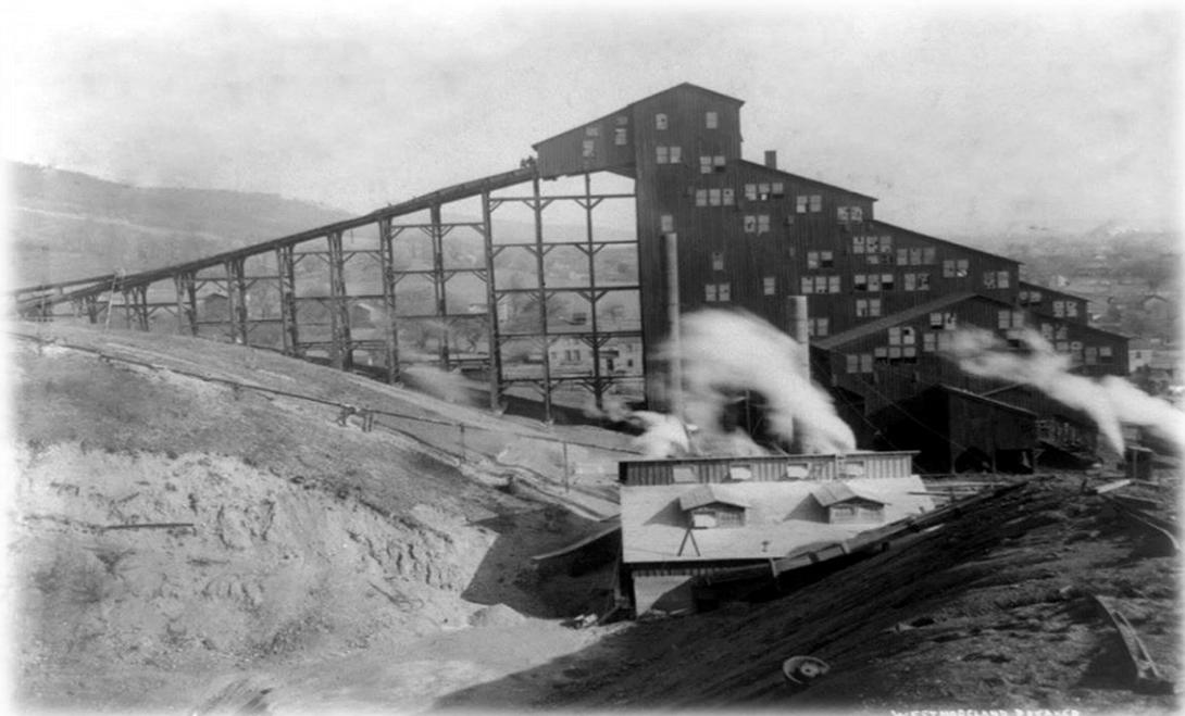
**Figure 5.** The Westmoreland Colliery during the early 20<sup>th</sup> century. Notice the small flume-like structure between in front of the breaker. It is possible that this contained flow from Novicki tributary.
