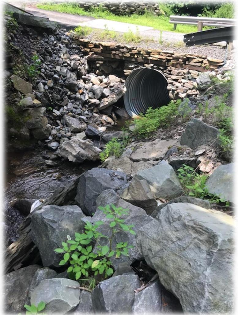
**Figure 14.** Degrading culvert headwall along West 8<sup>th</sup> Street. Notice the roadside bank is well armored while the landowner side is showing signs of degradation.
