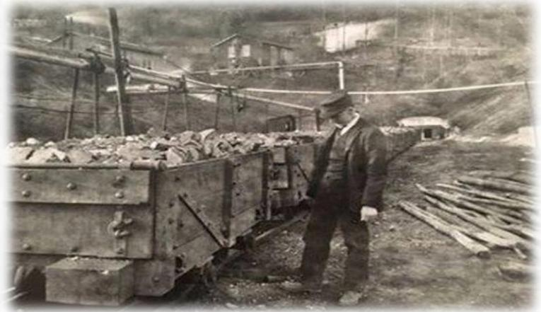
**Figure 7.** Mine entry to Westmoreland Colliery workings. The elevated structure on the left of the coal carts is the steel flume used to convey a portion of Novicki tributary.
