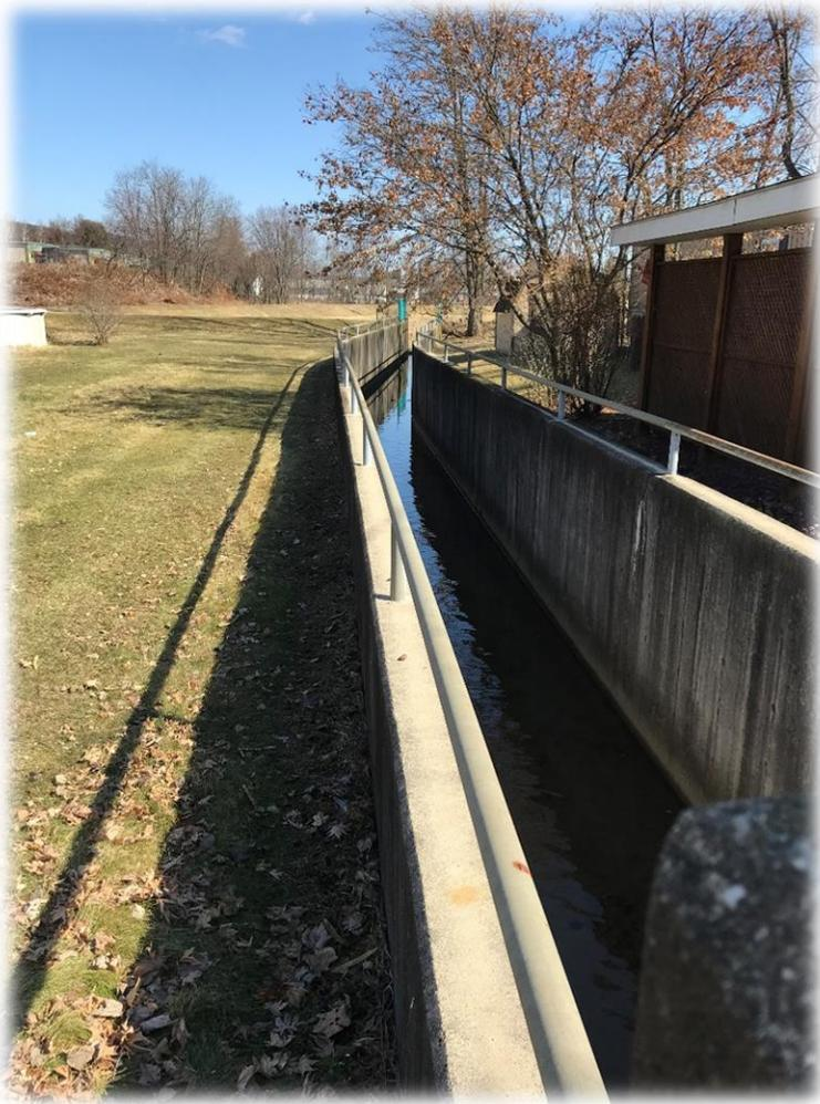
**Figure 17.** Seasonal flows occasionally fill the concrete channel that conveys surface water off of the Swoyersville pile and adjacent mountainside. Concrete lined channels characterize much of the lowland section of Abraham's.
