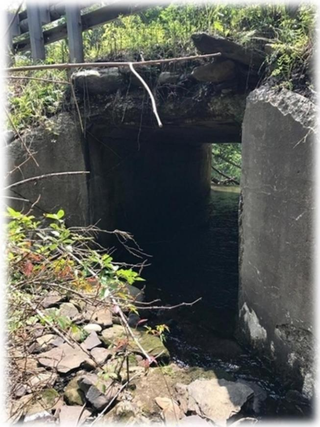
**Figure 12.** Dilapidated culvert where Mt. Zion trib flows underneath West 8<sup>th</sup> Street in The Hollow. This represents an extreme barrier to fish passage and significant infrastructure failure/flooding risk.
