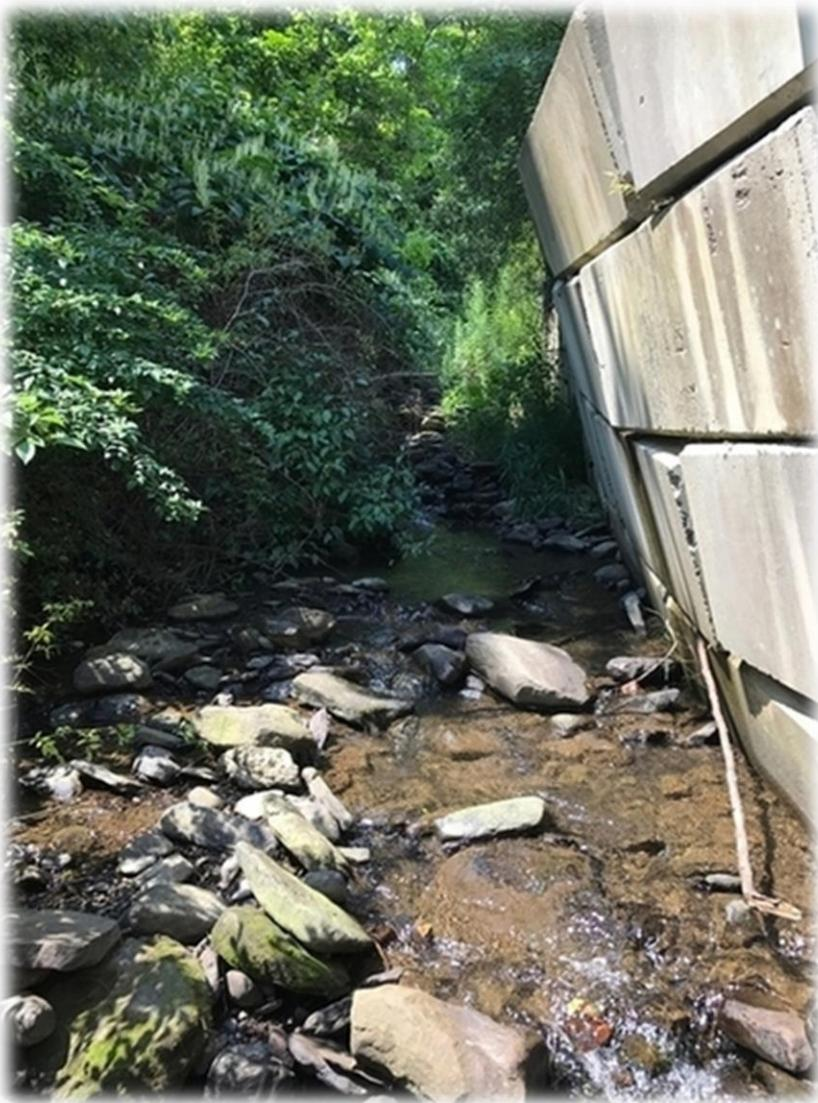
**Figure 13.** Wingwall on the verge of collapse in the West 8<sup>th</sup> Street section at Carverton Auto Sales. This culvert is in immediate need of rehabilitation to mitigate risk of flooding over West 8<sup>th</sup> Street.
