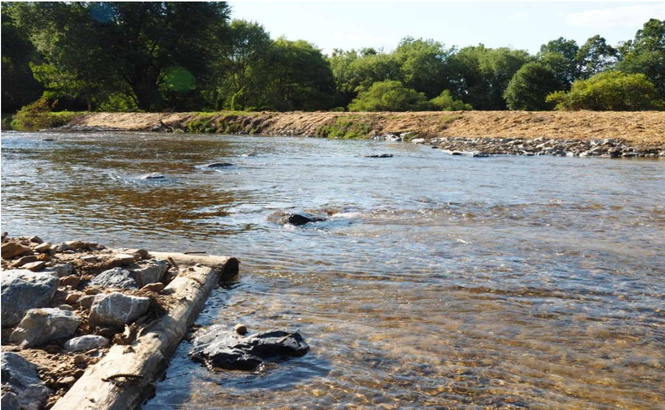
Placement of random rocks throughout the stream in the project area
