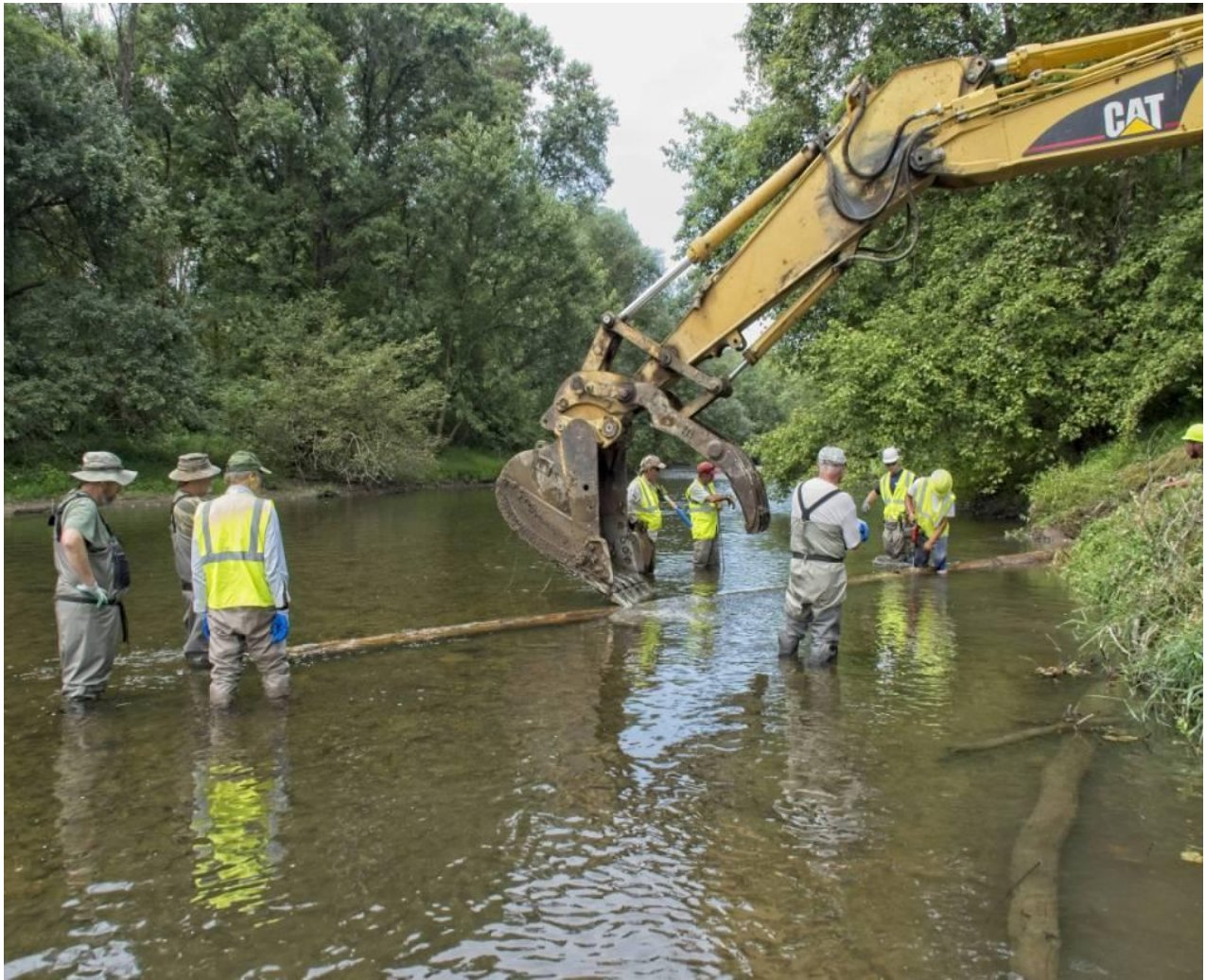
CVTU Volunteers building the first Log Framed Stone Deflector
