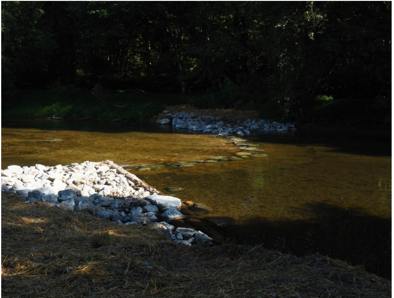
Completed J Hook Structure at the head of the stream channel
