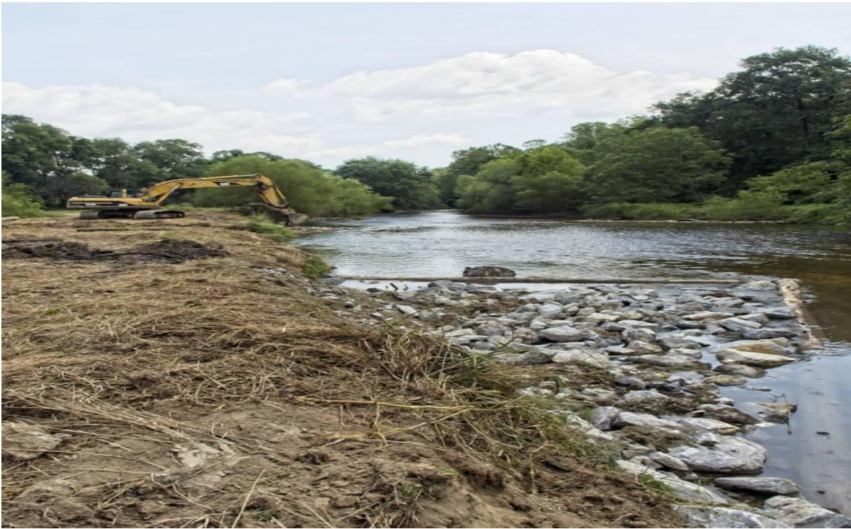
Backfilling the Log Framed Stone Deflectors
