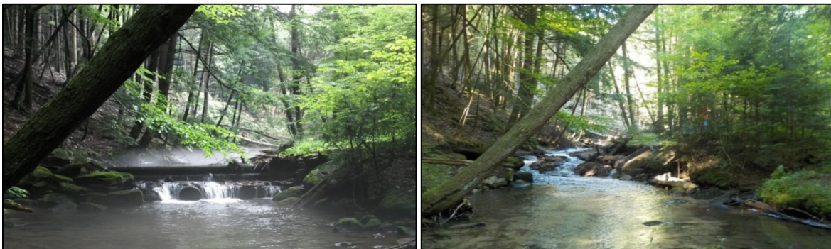
Johns Run before (left) and after (right) dam removal to restore passage to 4.75 miles of stream
