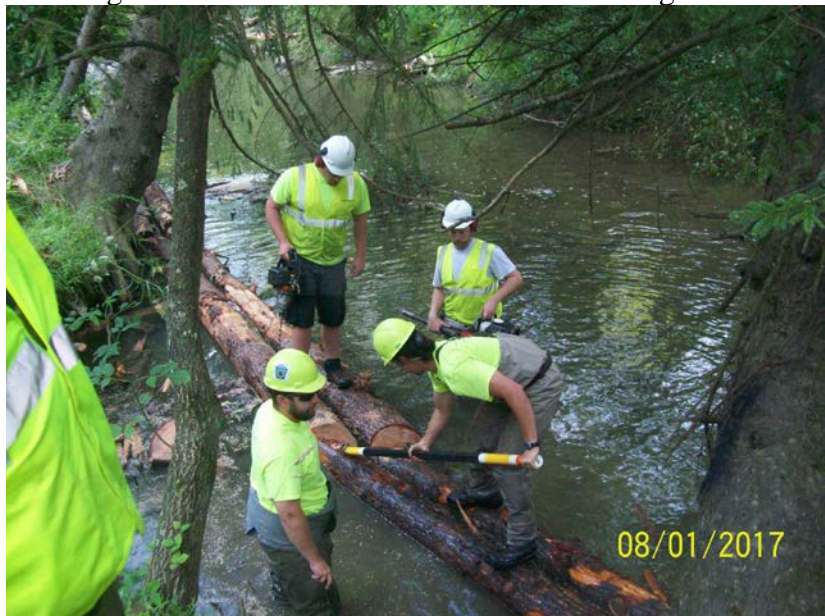
Mud sill #46 a very labor intensive area..
