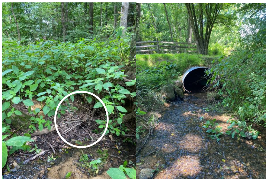
Figure 12. Showing inlets of culverts 5 and 6. Culvert 5 (left) has major constriction at the inlet and was mostly buried. The white circle on the left picture shows the relative area of where the culvert is being clogged. Culvert 6 (right) has physical barriers and little to no matching substrate covering the bottom of it.
