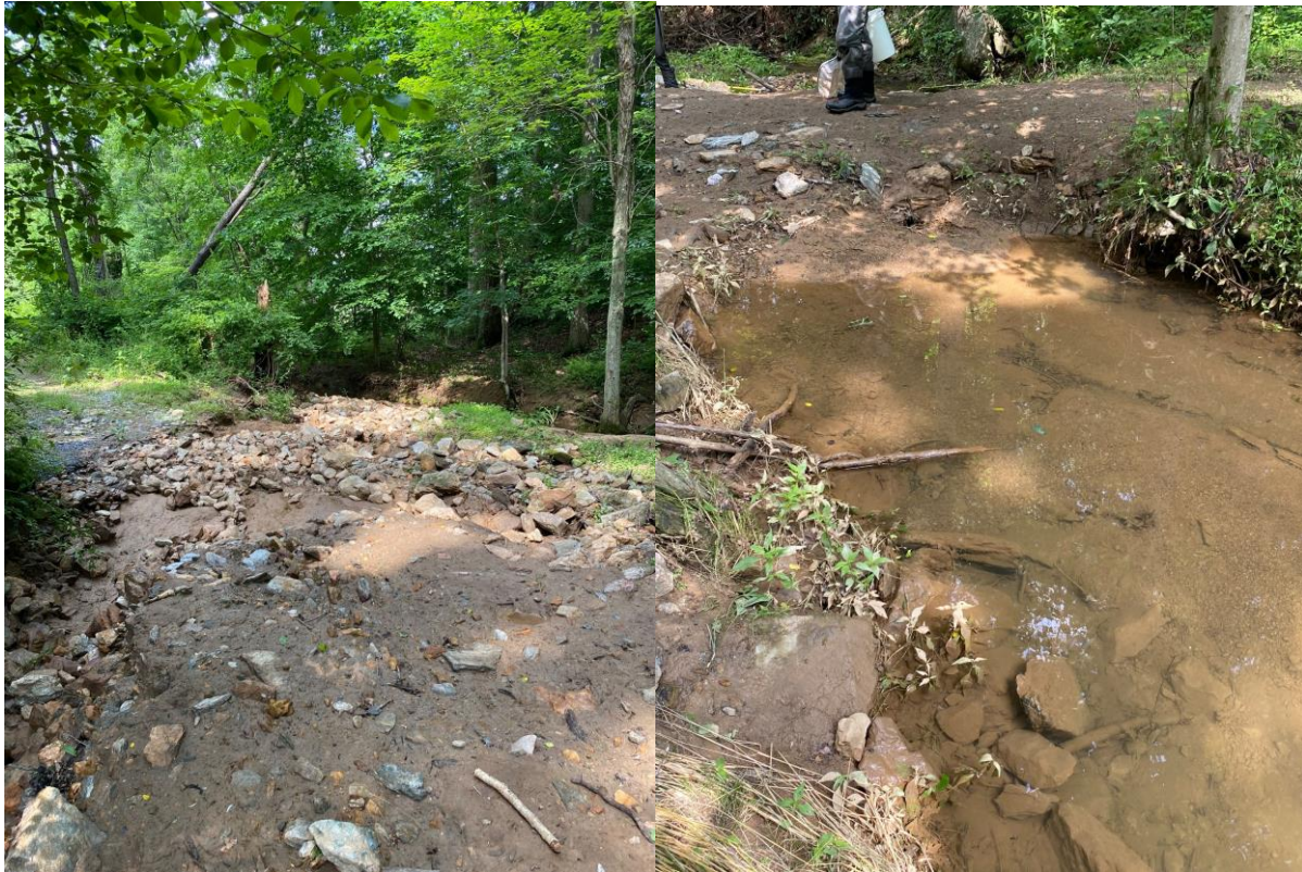
Figure 14. Left image shows the conditions following 7-inch rainfall event where the stream reached a level above bank full, bypassing culvert 5 and eroding township road (left). The right image shows culvert 5 inlet completely blocked following bankfull event.
