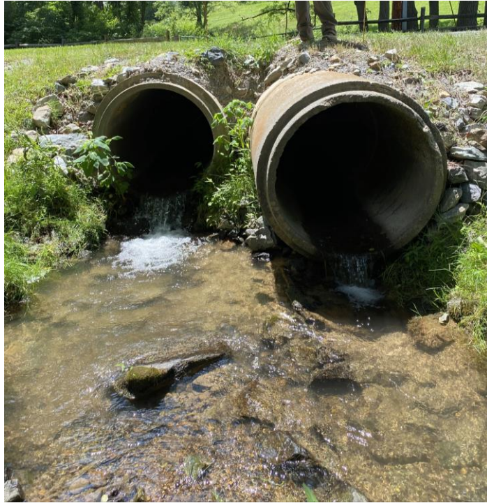
Figure 13. Depicts outlet of culvert 8. Freefall numbers were 1.18 and 0.66 tenths of a foot respectively.
