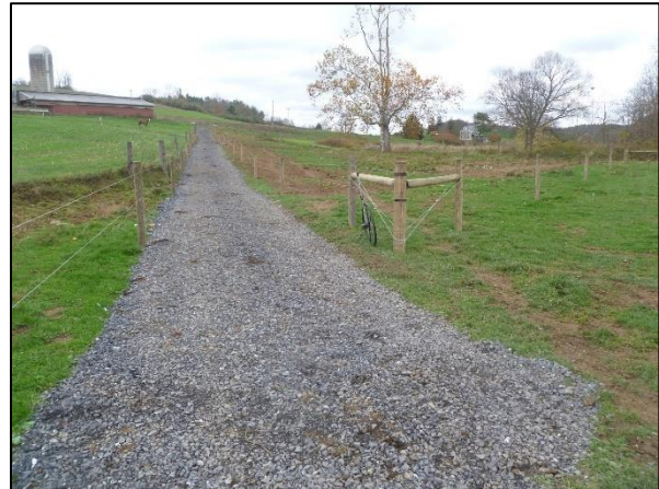
Photos 2-3. Before and after example of an NRCS cattle walkway stabilization project to improve soil health and water quality ( photos provided by James Steward ).
