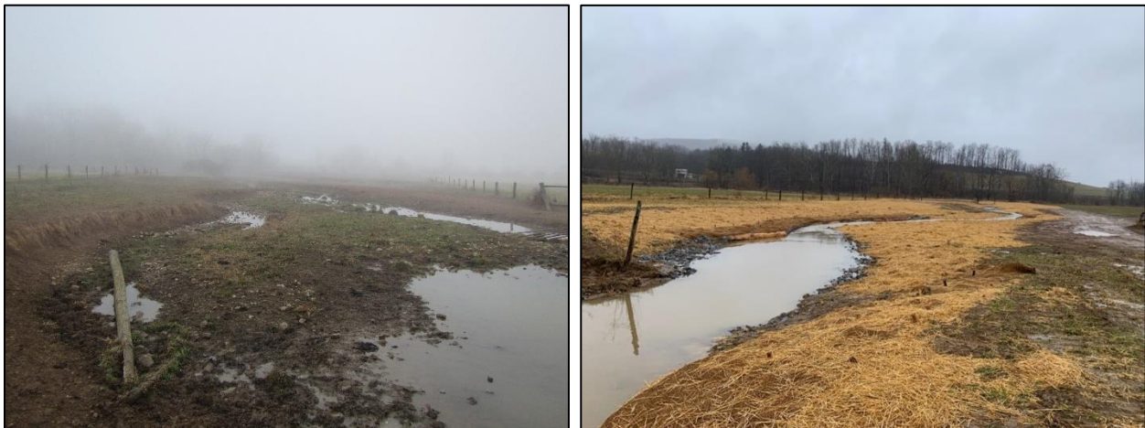
Photos 21-22. Before and after pictures from a stream restoration project along Shavers Creek, a comparable HQ-CWF stream to Standing Stone Creek, in Huntingdon Co. 2021.
