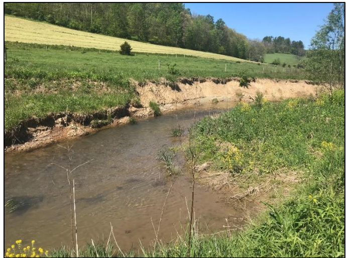
Photo 23. Example of eroding stream banks along Herod Run at site HR-01.
