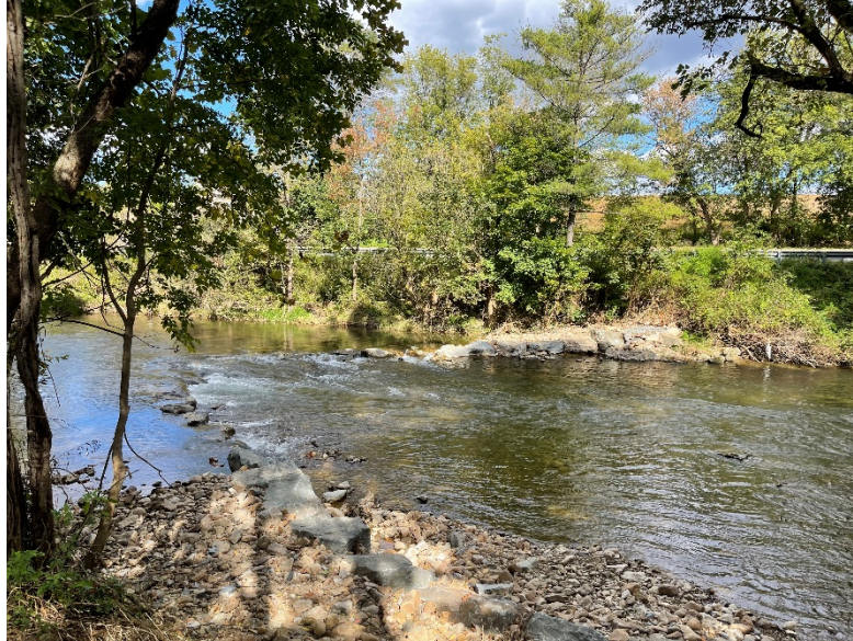
After photo of one of the 19 instream structures. Each structure creates a diversity of flow and instream habitat. A deep pool is forming downstream from the structure while creating more shallow, slower flow conditions along the stream banks for added habitat and stream bank stabilization.
