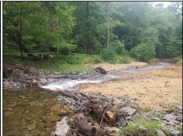
Final Clear Creek main channel after Phase I & II
