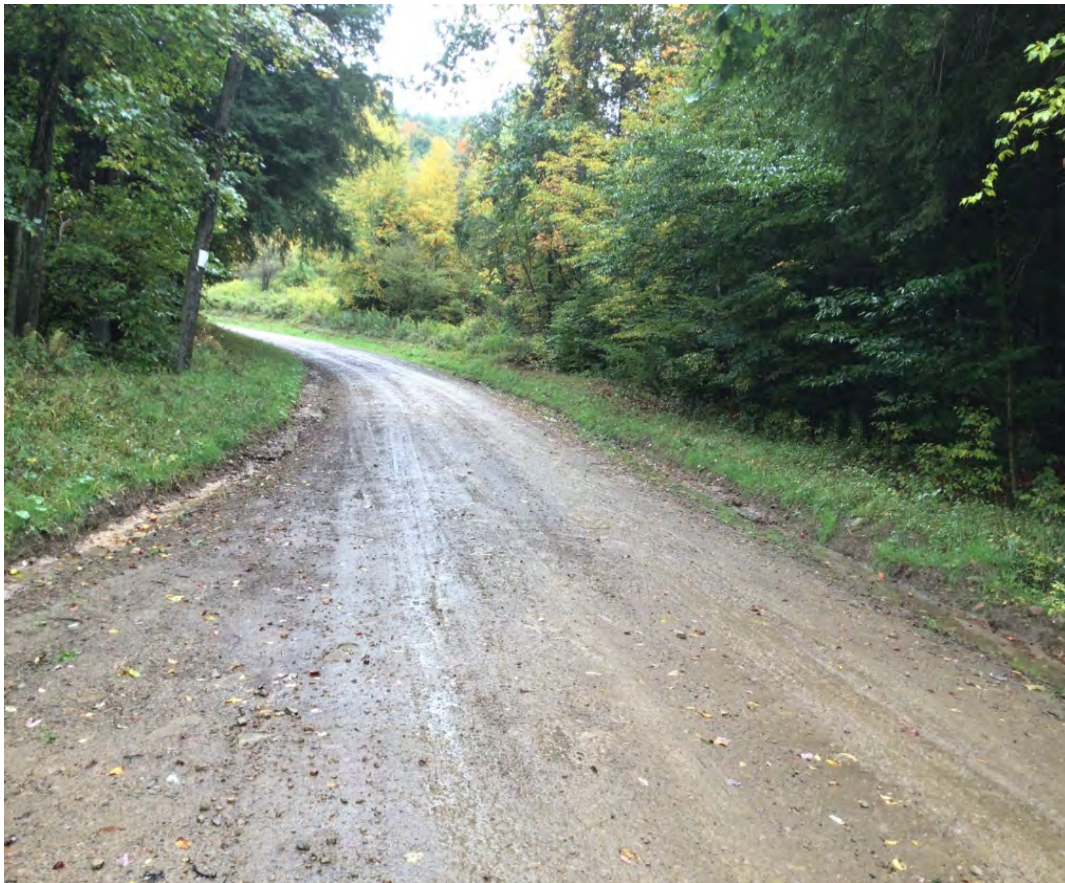
Photo 7: Runoff from dirt and gravel roads carry sediment and pollutants and when not maintained properly can negatively impact water quality and aquatic habitats.
