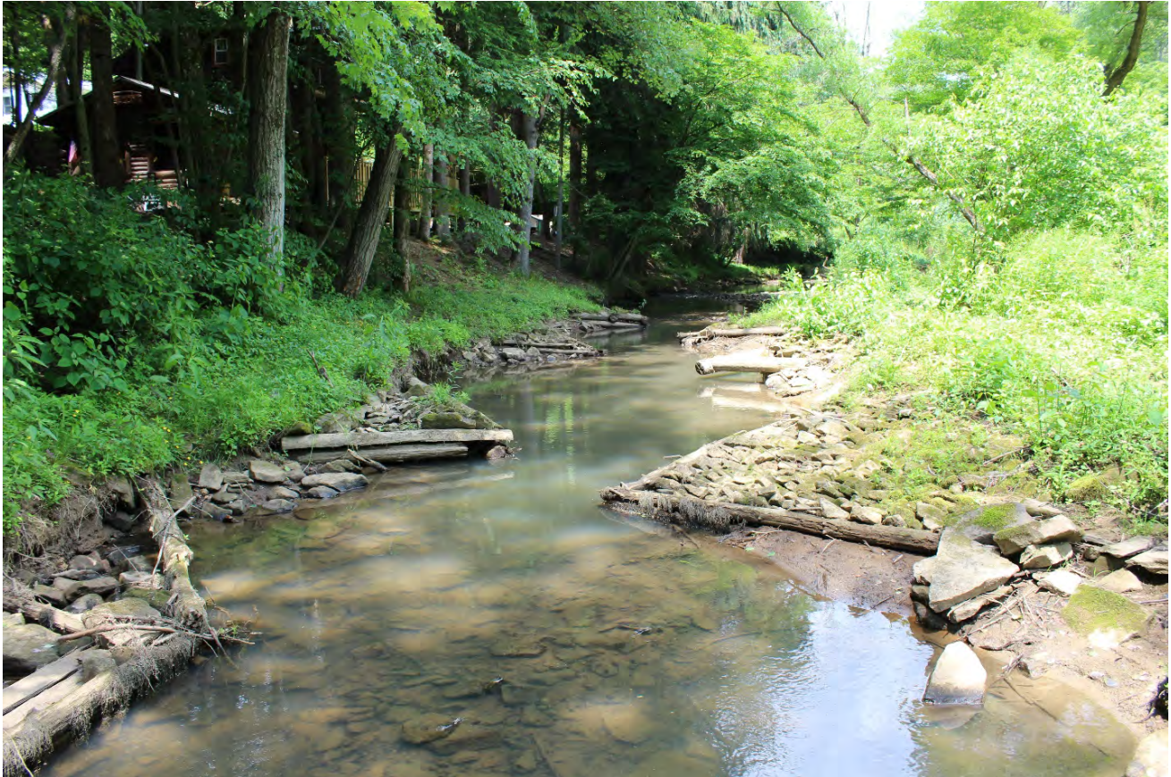
Photo 9: Antiquated aquatic habitat/stream stabilization structures on Big Run.
