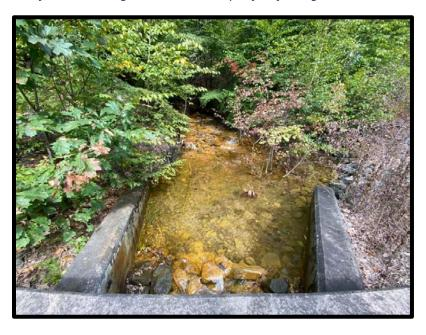
Figure 23. Concrete culvert carries Packer Air Shaft AMD discharge under railroad before dumping into Gardner Creek
