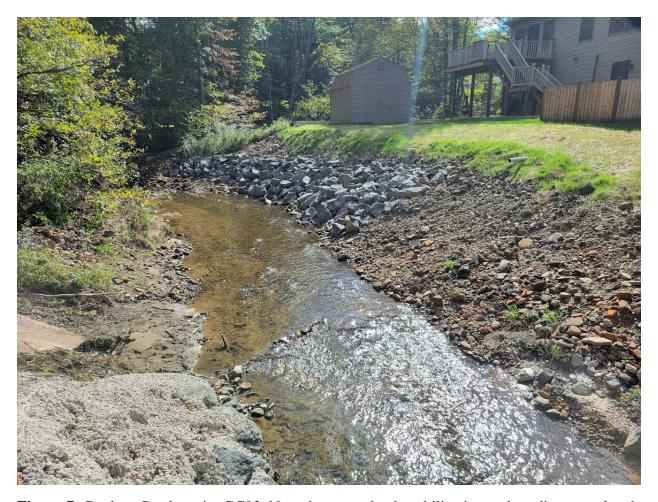
**Figure 7.** Gardner Creek at site GC03. Note the recent bank stabilization and grading completed during summer 2021 after heavy rainfall negatively impacted the area.
