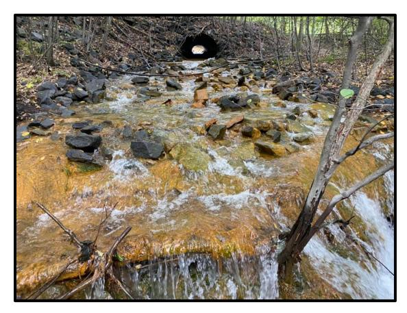
Figure 24. Looking upstream on the Packer Air Shaft AMD discharge thru the squashed corrugated metal pipe culvert
