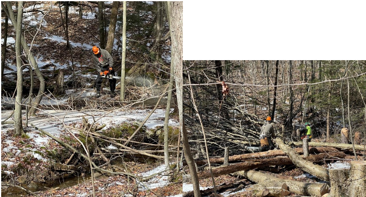
Photos 3 & 4: LWD addition on floodplain, side channel, and main channel along Water Tank Run (2022)
