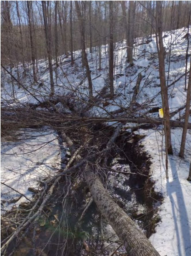
Picture 4. Chop and drop remediation used to slow velocity and assist in floodplain access for site depicted in picture 3.
