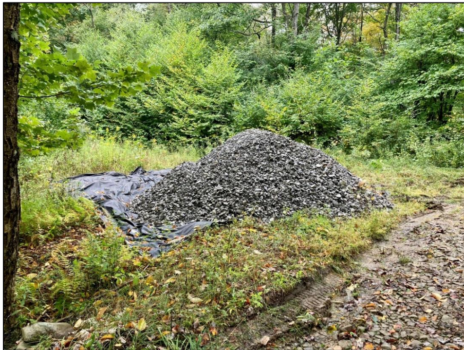
Geotextile fabric and limestone placement prior to construction of stabilized pad at Berkebile Run
