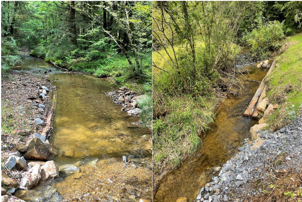
Photo 2. Mudsill on left side of photo
