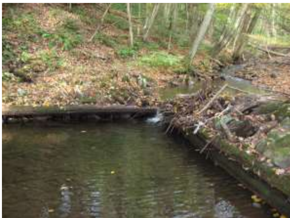
Wallacks Branch Burnt House site before
