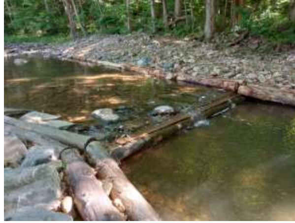
Bobs Creek at Ickes site after restoration
